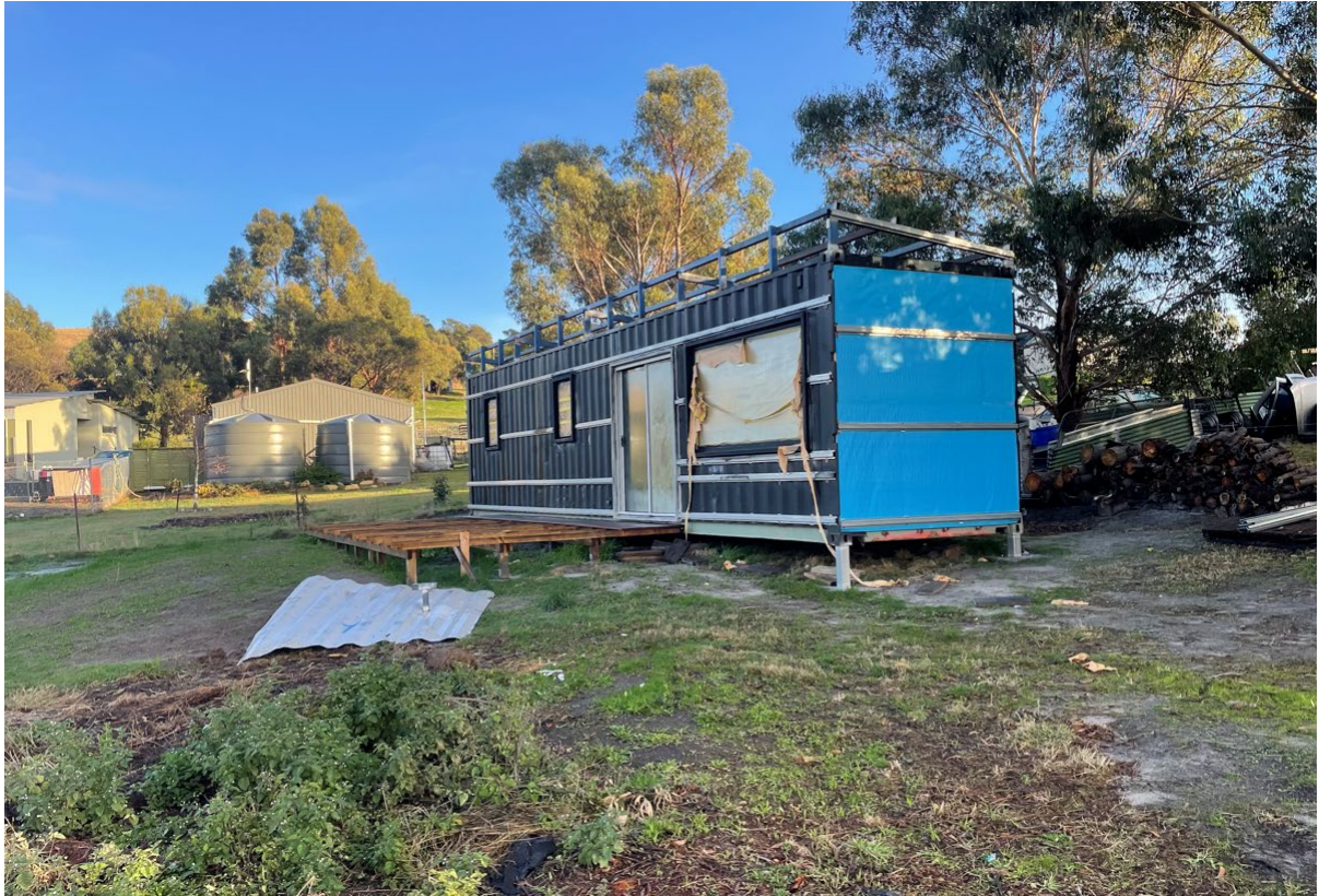
Photo 5: Field photo taken showing existing shipping container to be converted into a Class 1a ancillary dwelling.
