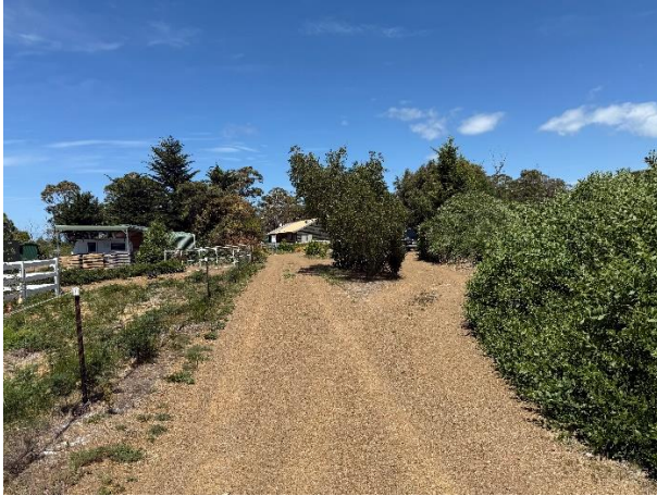
Figure 5 – (part of) existing access to Lot 2
