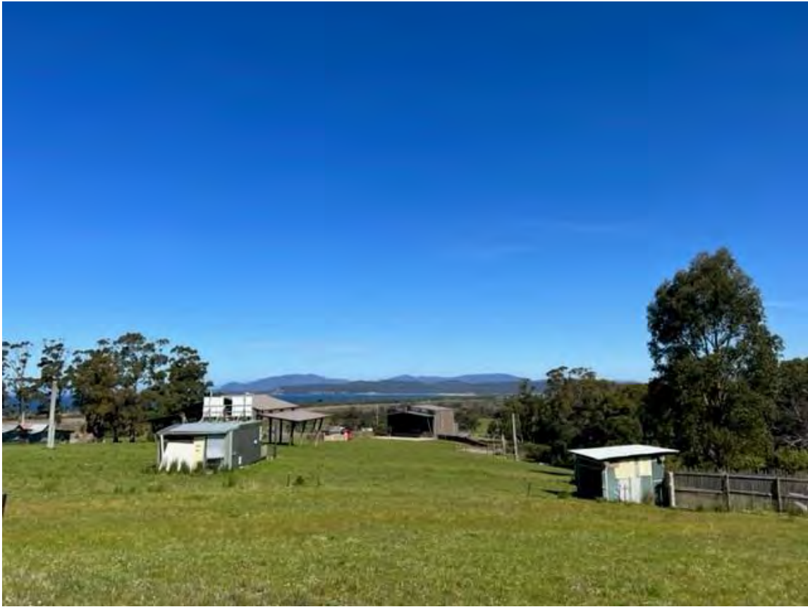
Figure 10 - Existing structures on the proposed Lot 3
