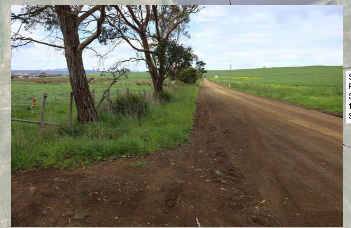
SIGHT LINES SOUTH FROM PROPOSED LOT 1 ACCESS SIGHT DISTANCE EXCEEDS 175m (80KM/H VEHICLE SPEED TSD-RF01)
