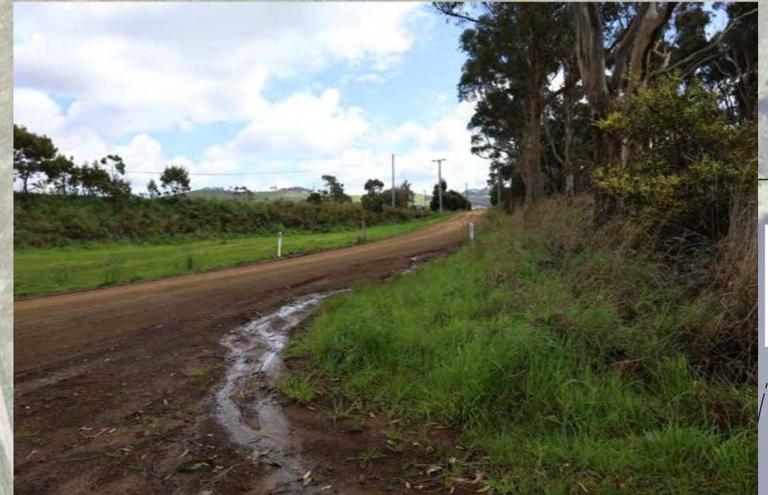
SIGHT LINES NORTH FROM PROPOSED LOT 1 ACCESS SIGHT DISTANCE EXCEEDS 175m (80KM/H VEHICLE SPEED TSD-RF01)
