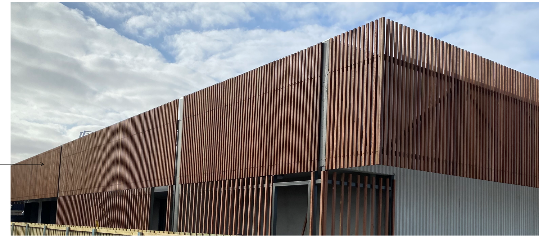
TIMBER SLATTED SCREENING FACADE ON PROPOSED BUILDING AS BUILT. NEW FRONT GATE AND FENCE TREATMENT TO MATCH THIS TIMBER SLATTED SCREENING.
