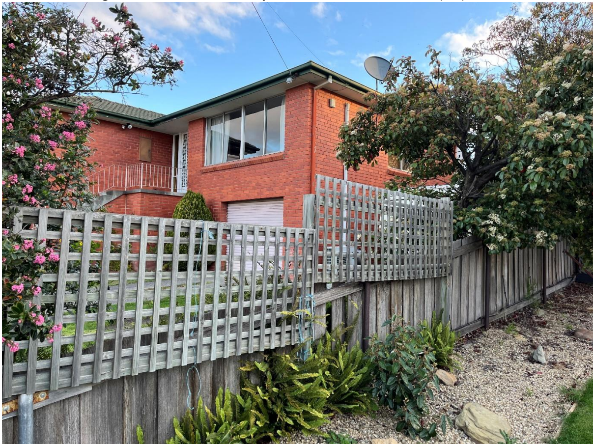
6 Lake Vue Parade showing fencing and planting on the boundary.
