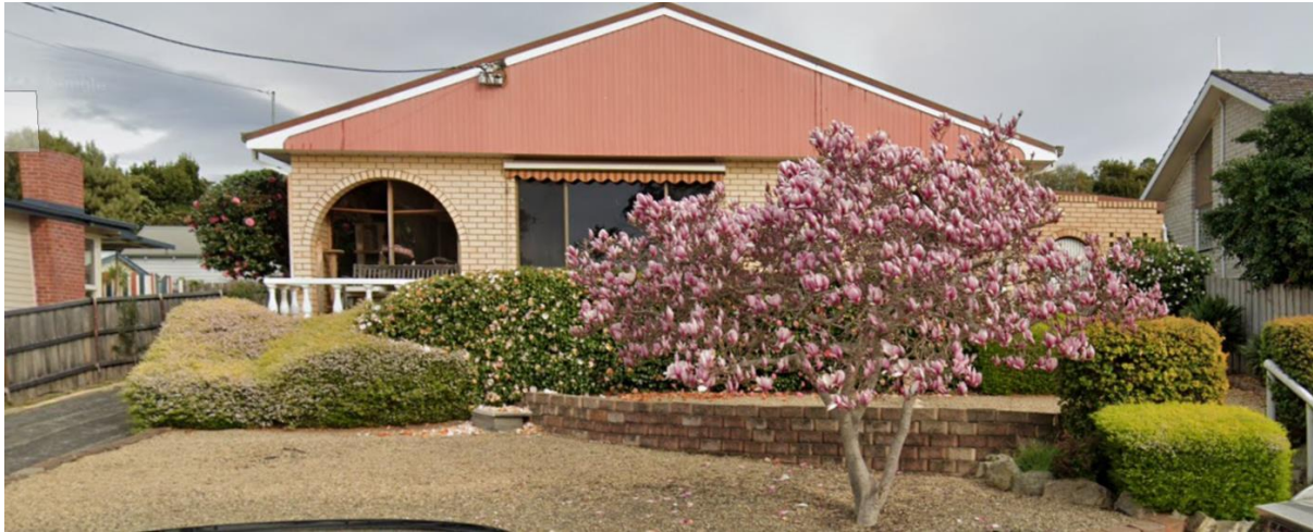
16 Lake Vue Parade, which has a masonry wall extending through to the boundary on the righthand side of the house.
