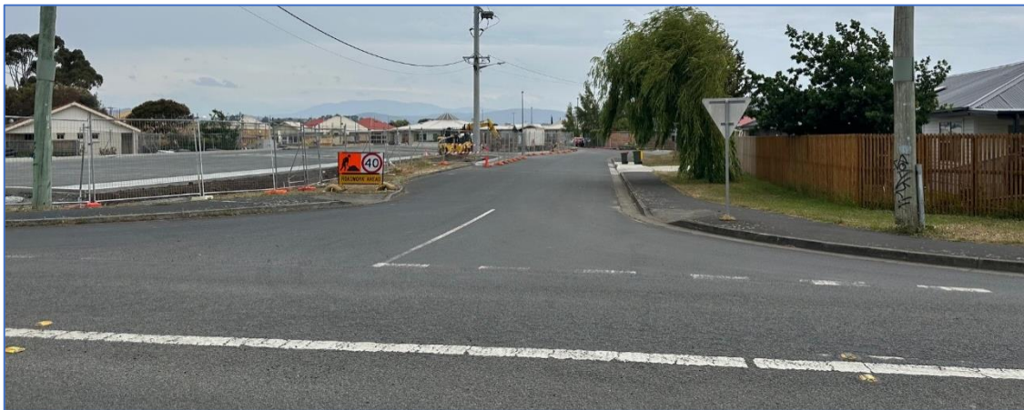
Photograph 5.2 – Arthur Street and Taylor Drive junction
