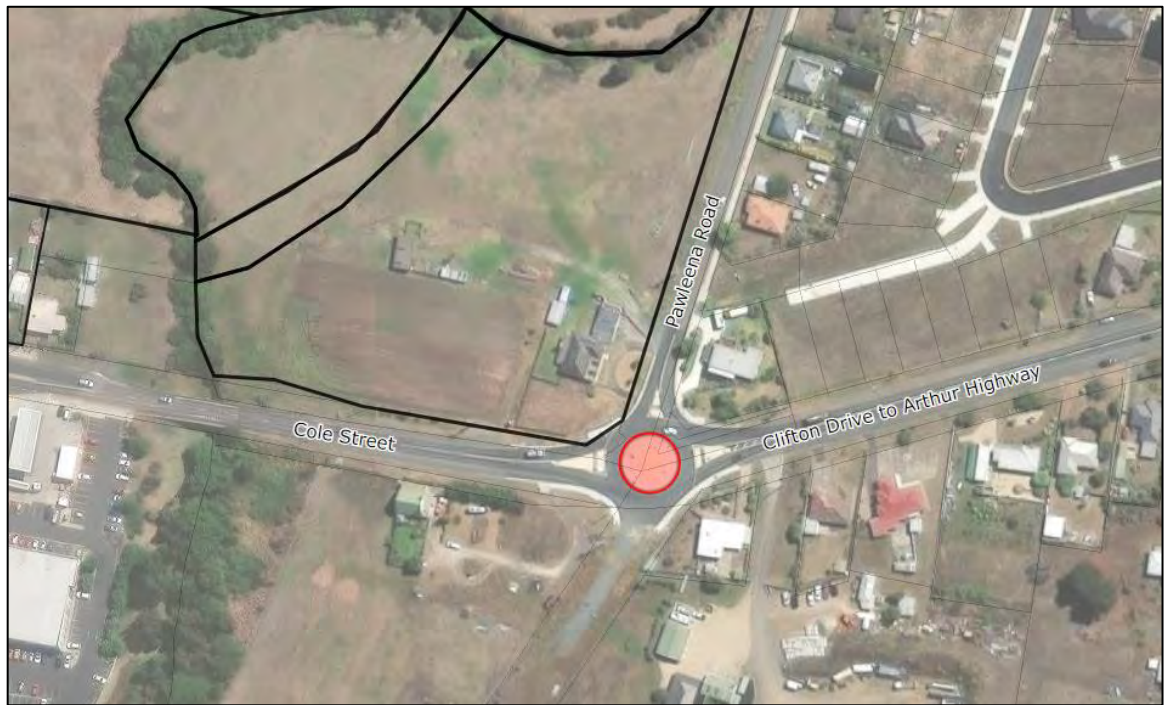
Figure 7: Aerial image illustrating the completed roundabout (indicated in red) (source: www.thelist.tas.gov.au © State of Tasmania)
