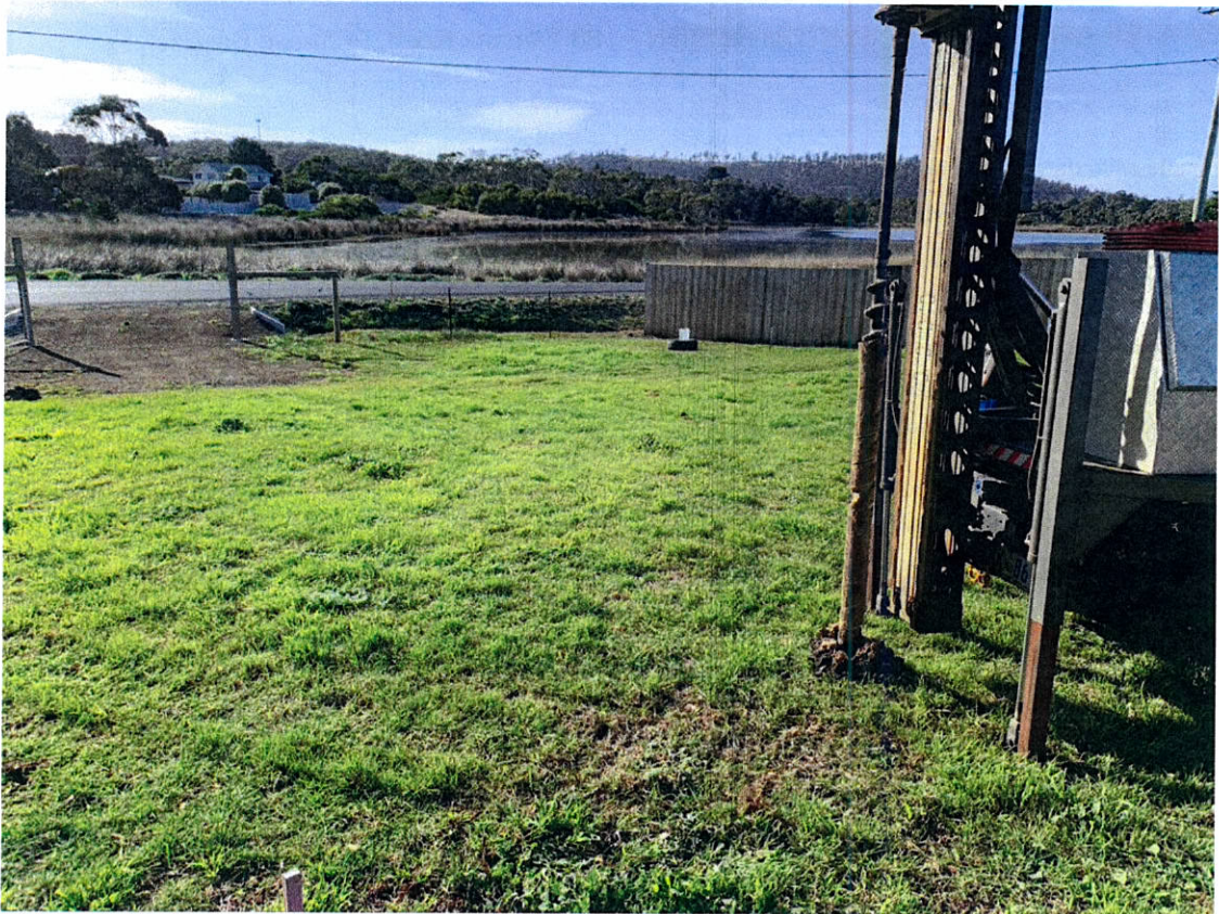
Plate 2 – Test Hole #3 – Looking to the northeast from the proposed LAA.
