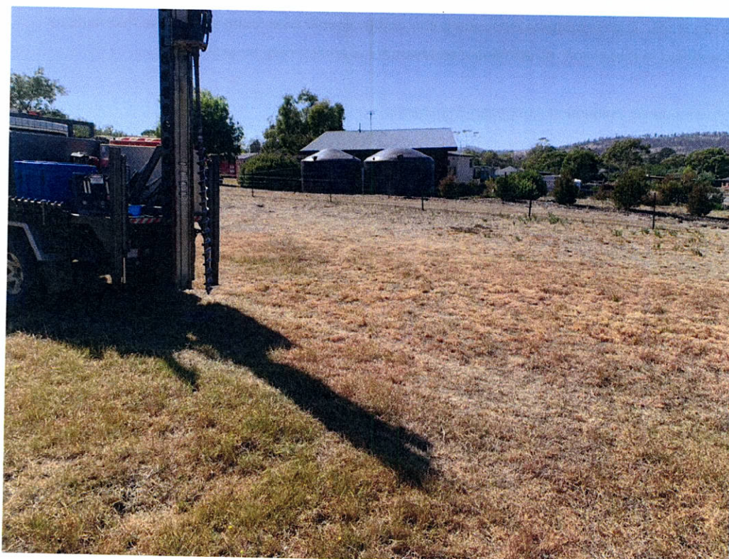
Plate 2 – Looking across-slope to the northeast (Test Hole #1).
