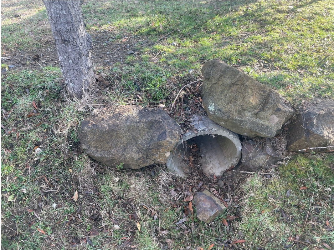
Figure 8. Culvert under footway (24 June 2024)
