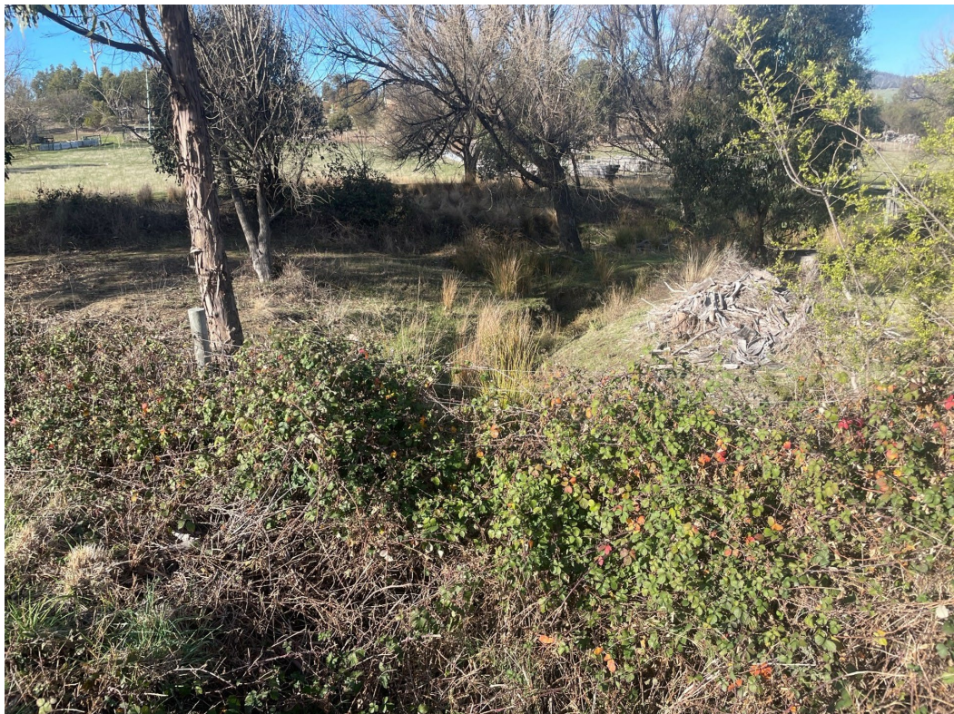
Figure 11. Open drain on eastern side of Ryans Lane facing south from highway (24 June 2024).
