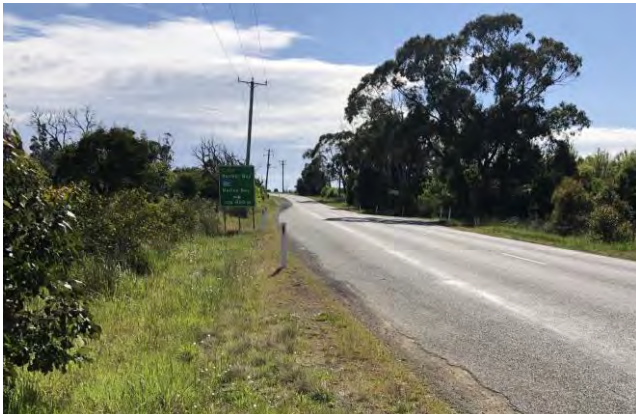
Figure 22 – Looking left along Arthur Hwy from proposed access
