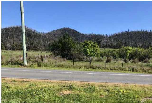
Figure 15 – Elevation view of the future road junction site.
