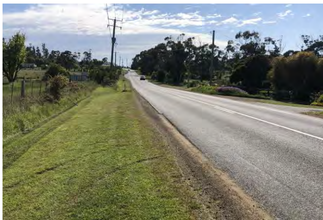
Figure 12 – Looking left along Arthur Hwy from future road
