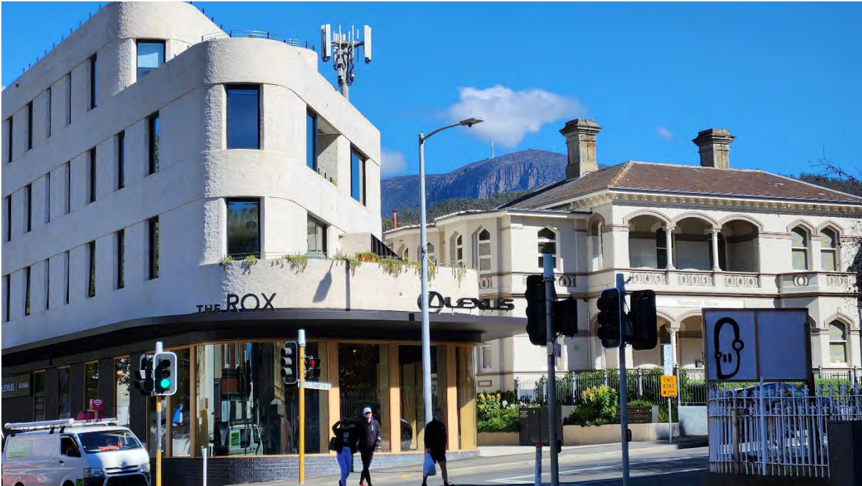
Figure 2 A mid-rise apartment in Hobart (source: ERA)
