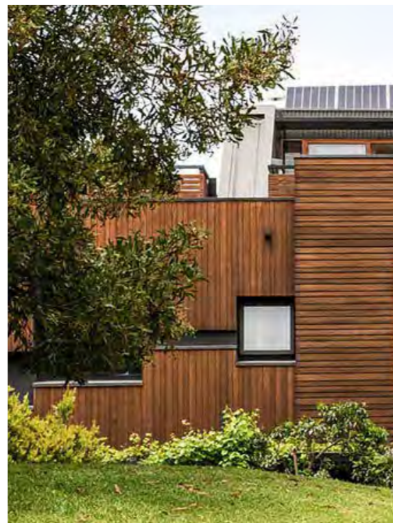
Timber battens provide vertical and horizontal expression and respond to natural settings.
