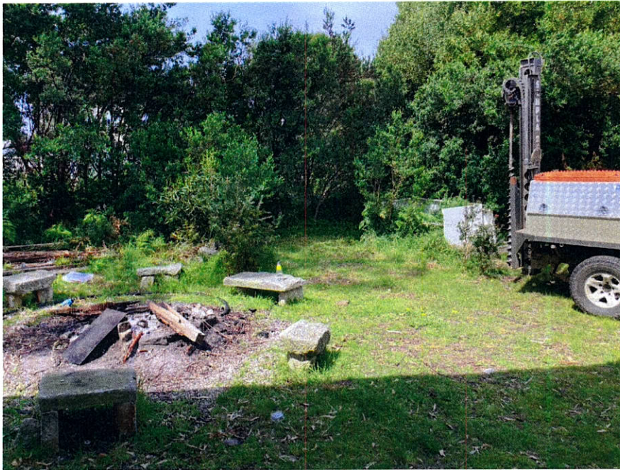
Plate 2 – Lot 1. Test Hole in the proposed LAA - Looking to the northeast.
