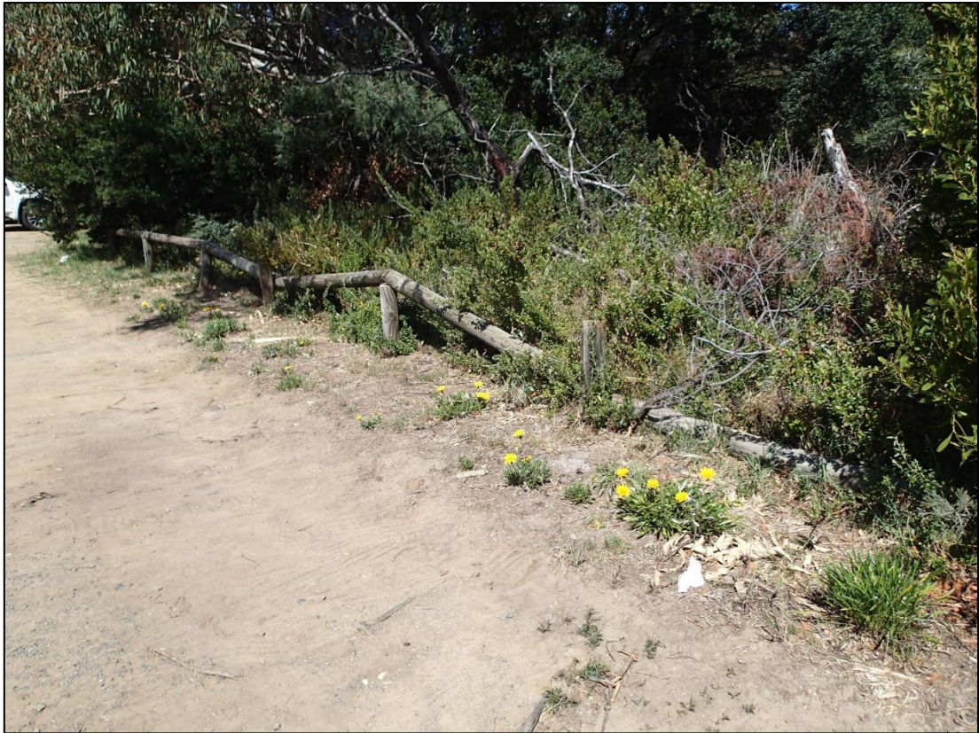
Plate 11: Fence along edge of parking area is in disrepair and overgrown with vegetation.
