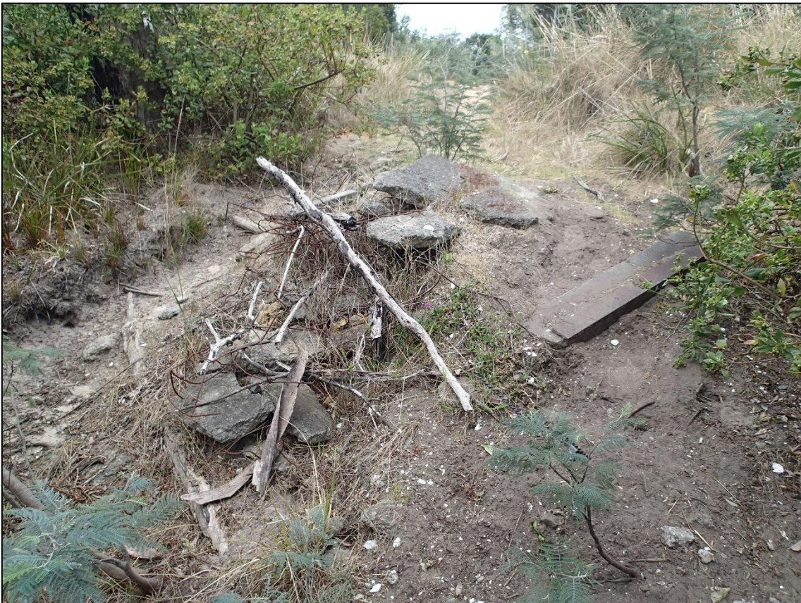
Plate 23: Building rubble along existing track should be removed for public safety.
