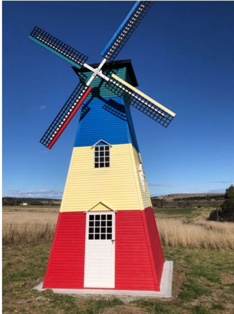
Figure 3 – Decorative Windmill Structure (7 metres in height)
