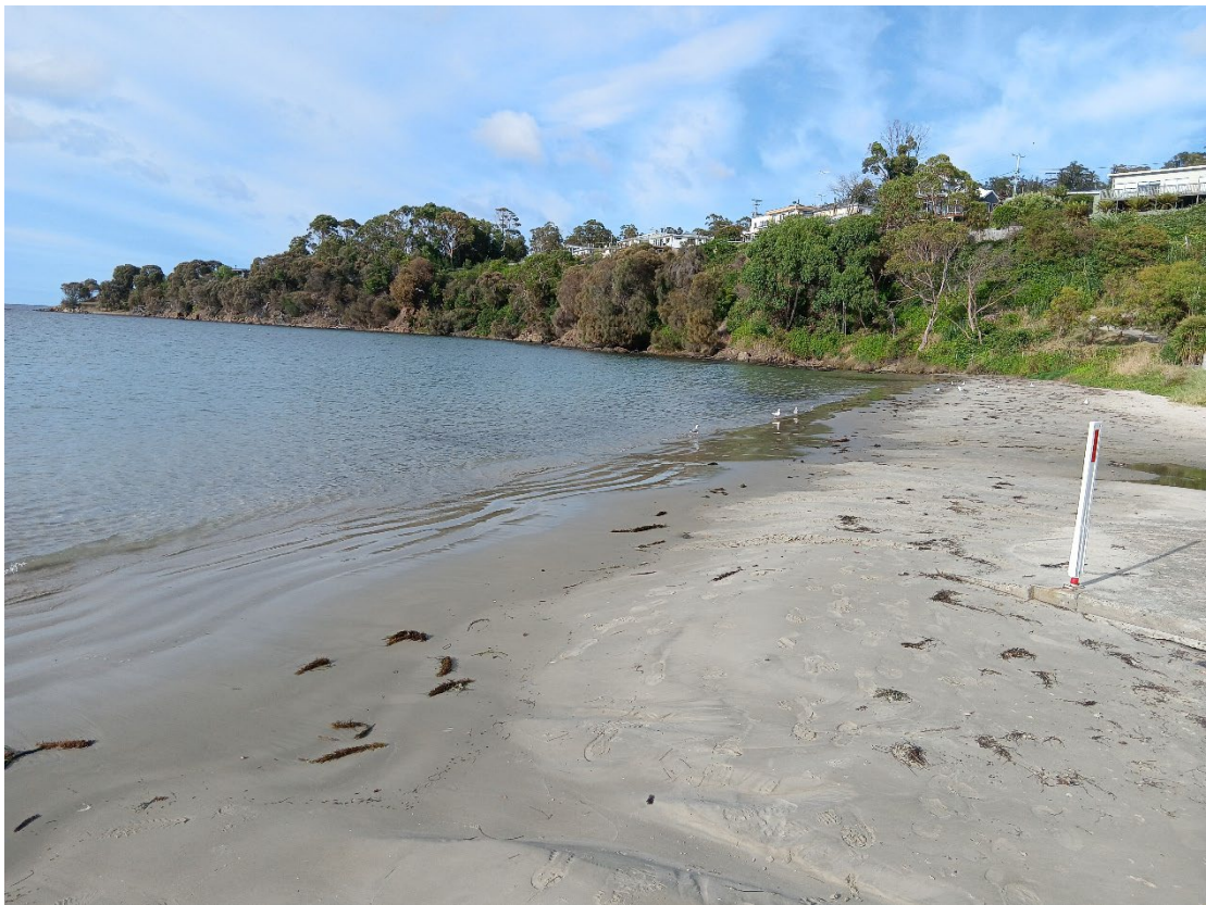
Seepage running onto Primrose Beach near the boat ramp.
